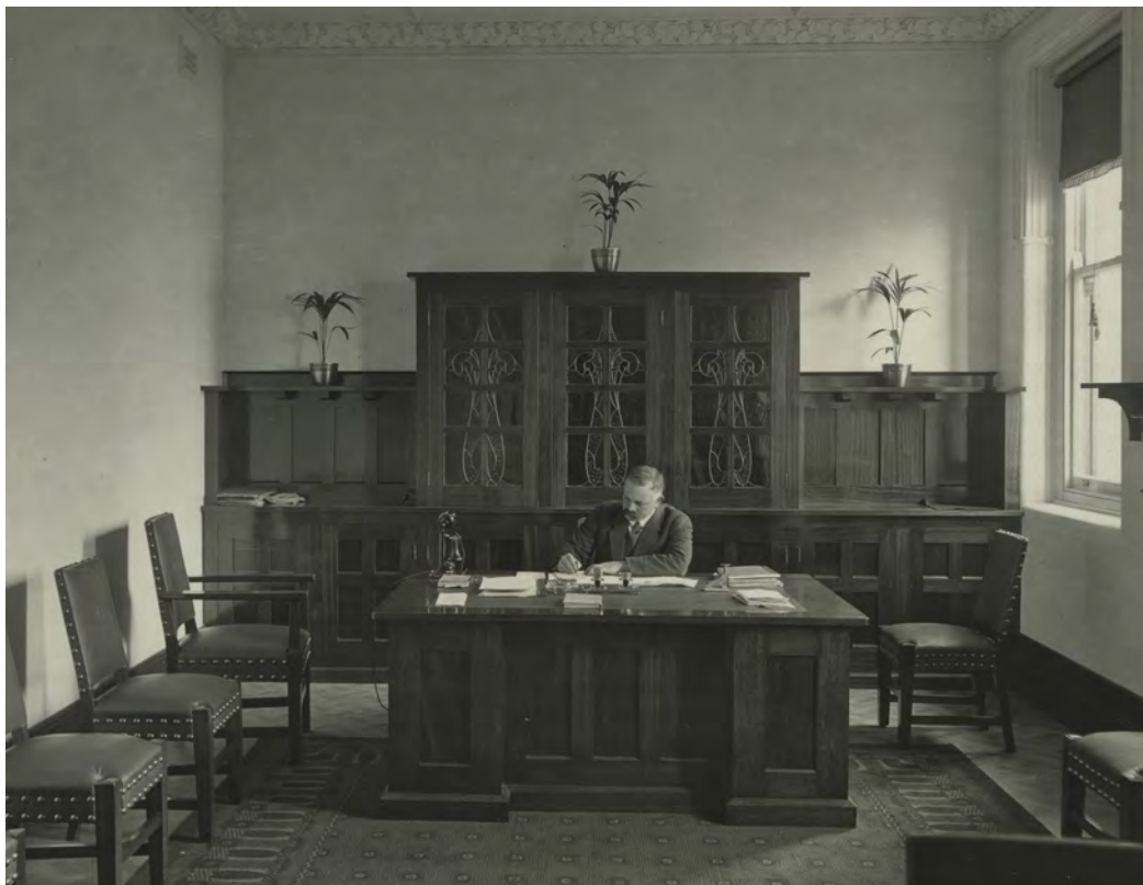
Figure 20. Town clerk's office on the ground floor, 1917 (GRS 2009/3873 Geelong Heritage Centre)
