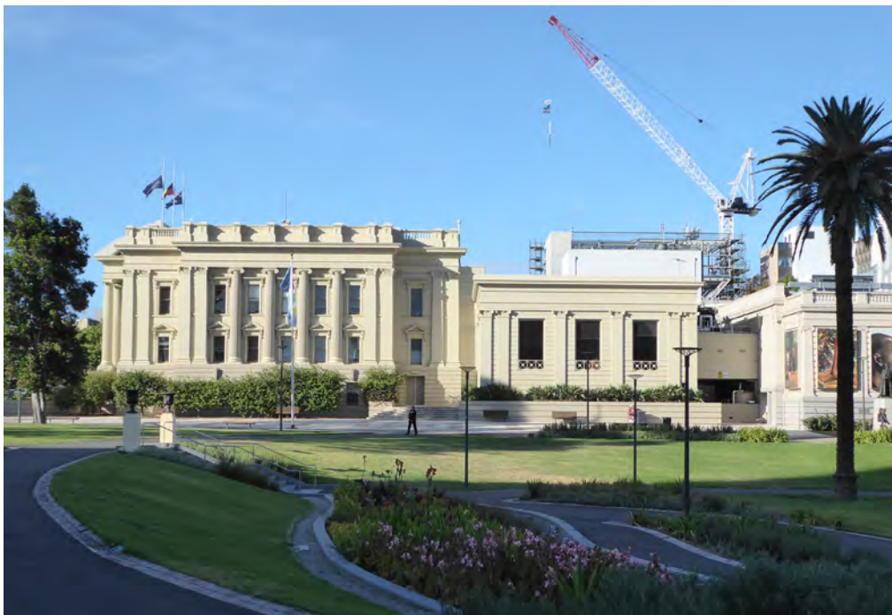
Figure 32. North elevation viewed from Johnstone Park
