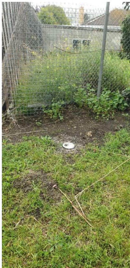
Photograph C.10: R-LFG-08 installed location (Rotary Centennial Park)
