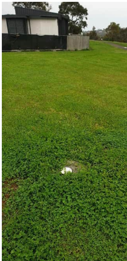
Photograph C.4: R-LFG-02 installed location (Rotary Centennial Park)
