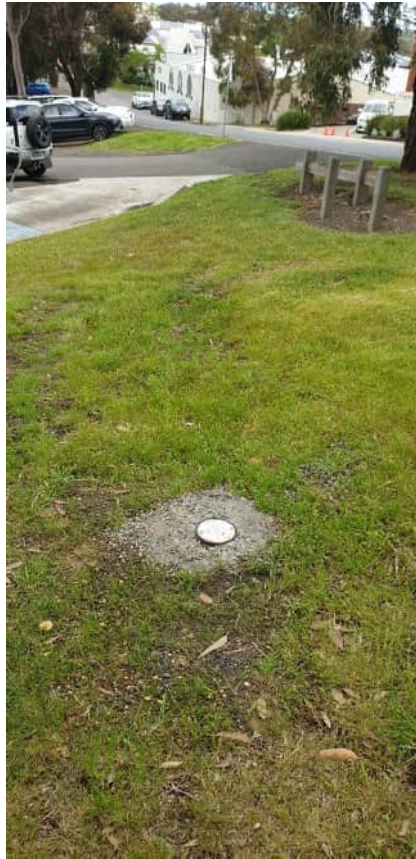
Photograph C.23: N-LFG-03 installed location (Newtown closed landfill)
