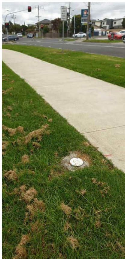
Photograph C.16: M-LFG-01 installed location (Marnockvale closed landfill)
