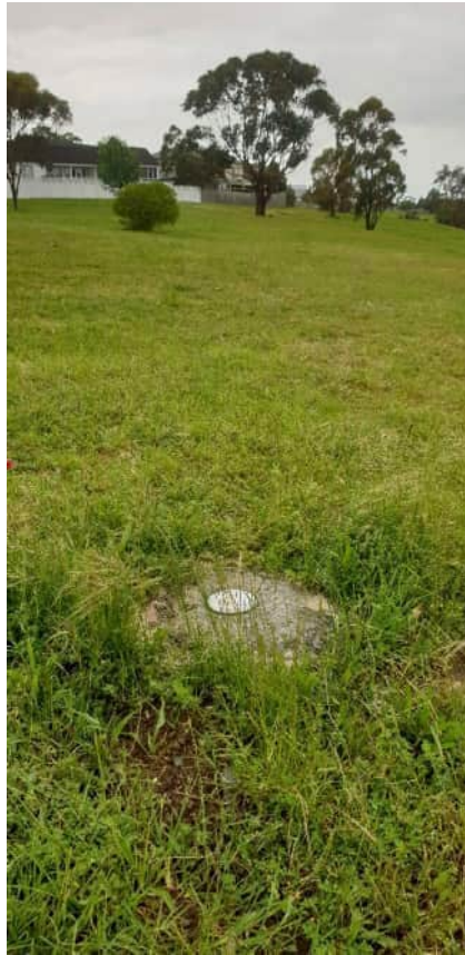
Photograph C.9: R-LFG-07 installed location (Rotary Centennial Park)
