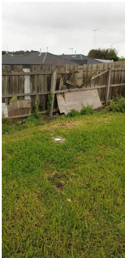
Photograph C.8: R-LFG-06 installed location (Rotary Centennial Park)
