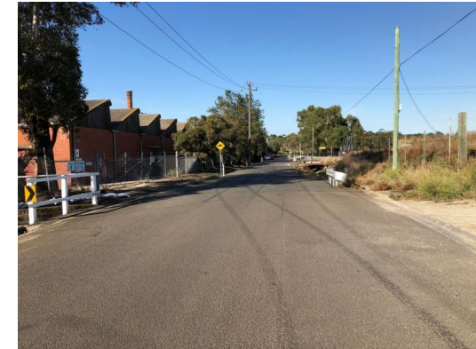
Bridge Road – drains present major hazard to vulnerable road users
