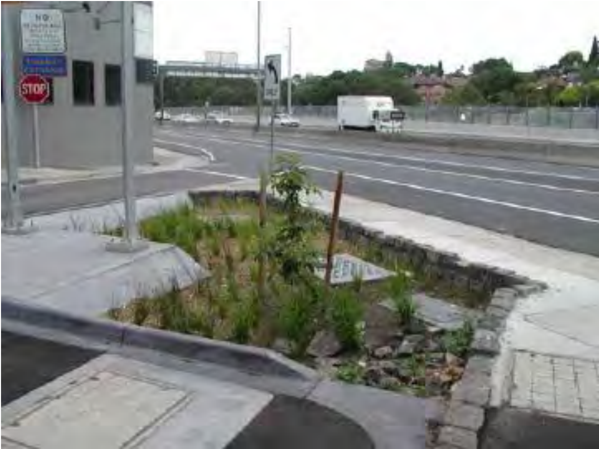
Figure 6.10 Streetscape raingarden (sourced from WSUD Engineering Procedures: Stormwater, Melbourne Water)
