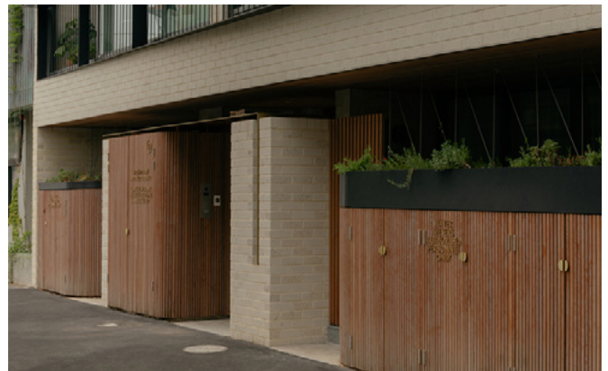
Napier Street, Fitzroy Services are concealed by integrating into the architectural design of the ground level, enhancing the street edge with visual interest through high quality finishes.
