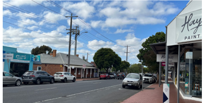
Isabella Street and Pakington Street intersection Looking to the south towards former Harp Inn. The street interface and character is eclectic with a variety of frontages including verandahs, awnings and exposed facades.
