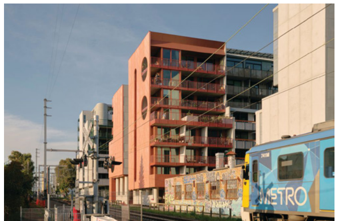
Nightingale Leftfield, Brunswick Located adjacent to the railway line and receiving the western sun, the building utilises the constraints to provide a podium that is textured, punctured with openings of different shapes and sizes to break the continuity and dominance when viewed from a distance.
