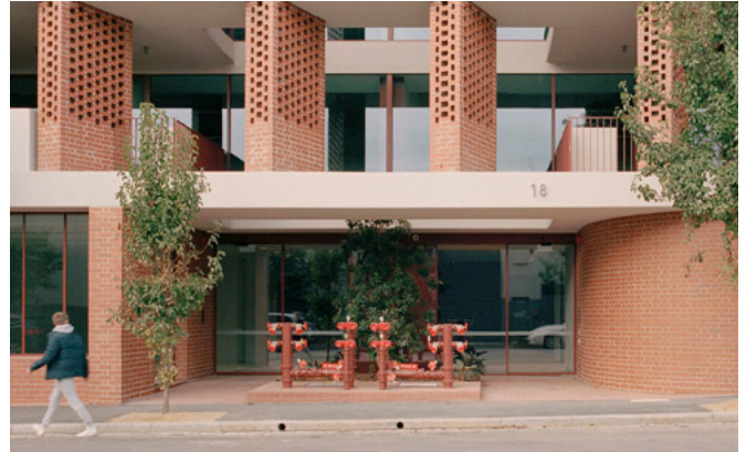
Napier Street, Fitzroy Services are visible but integrates with the overall design of the building and appears as a distinctive feature element.
