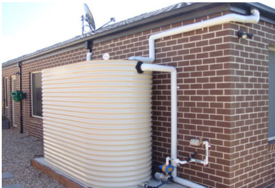
Figure 17: Typical Onsite detention system.
